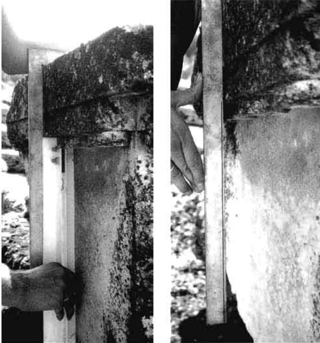
1. Architrave block, from corner. Measuring the angle. The line drawn on the metal square (right) enhanced. (Photographs by P. Pakkanen, 1995.)
